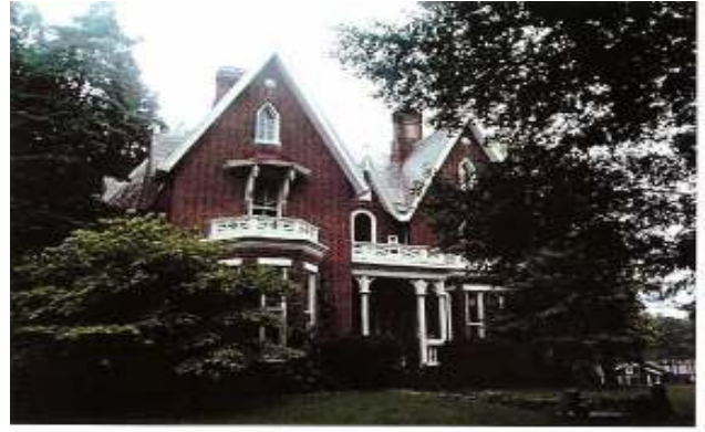
THE ANCHORAGE – This Gothic Revival villa gave Anchorage its name. Built in 1868-69 by riverboat captain James Goslee, its brick construction with carved wooden verge boards, 12-foot ceilings, and a steep roof pitch give it an extremely vertical look.
