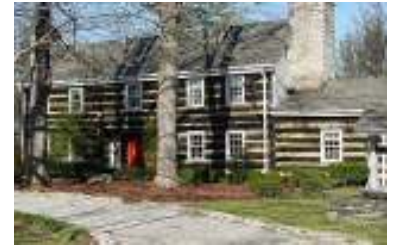
NEWLAND FARM was bought and developed by J. L. Shallcross. His home was constructed of cherry logs with stone chimneys. The house was originally a double log cabin with a covered dogtrot. A well still remains in the front yard. The home is one of several remaining log structures in Anchorage, and makes a significant contribution to the architectural and historic character of the City.
