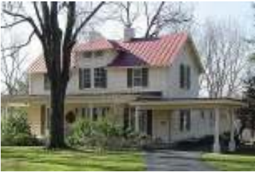
The JAMES F. WALKER HOUSE was built in the 1860's. This three-bay, two-story frame house has the front entrance placed in the central bay and is flanked by sidelights. A one-story porch, supported on modest columns, spans the façade and curves around the south side. A porte-cochere was added on the north side,
